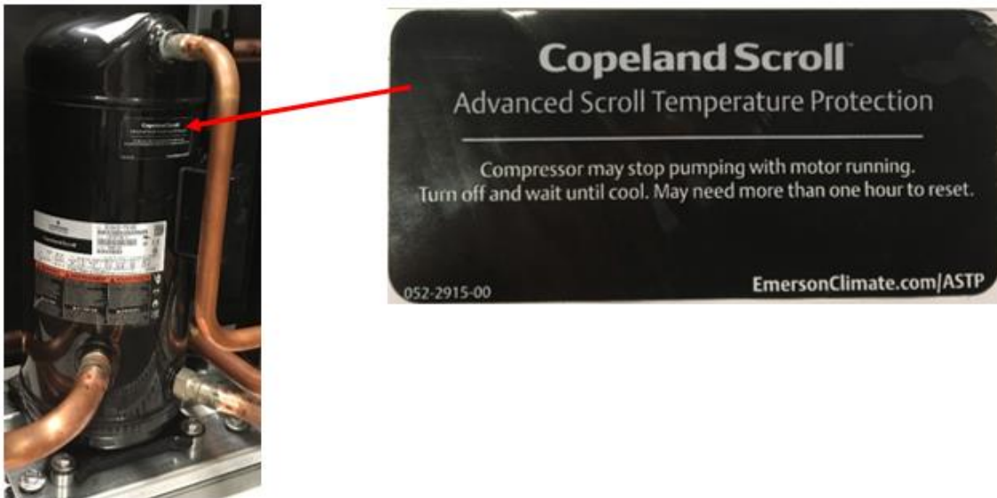
Figure 20: Advanced Scroll Temperature Protection (ASTP)
